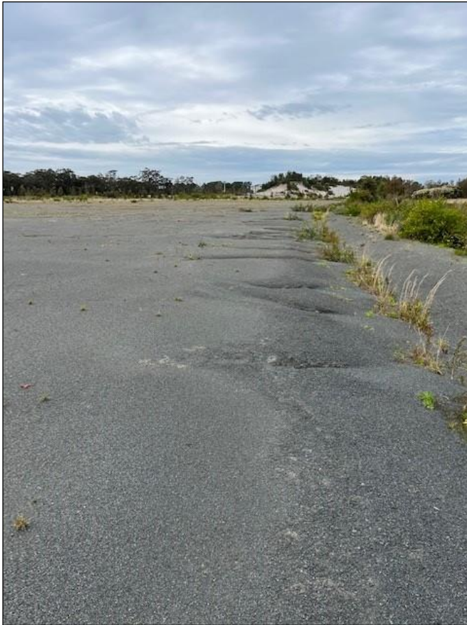
Figure 10: Localised erosion in the southern portion of the site (15 September 2022)
